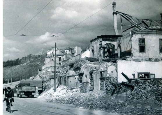
Picture 19 - Demolition of the Đumrukana building
