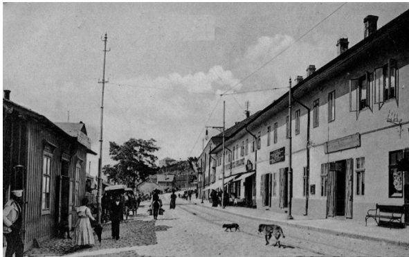
Picture 16 - the "Kragujevac" Hotel, early 20th century
