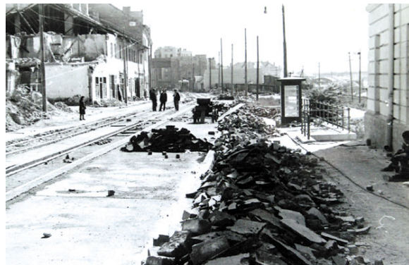
Picture 17 - the "Kragujevac" Hotel building - demolition
